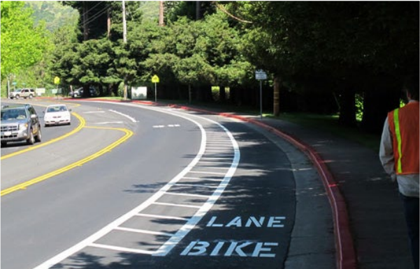
Painted Buffered Bike Lane
