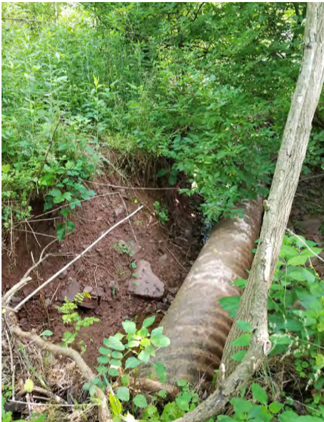
The unnamed stream exhibits signs of erosion along the culvert pipe at the low point of the site, likely from high volumes of stormwater runoff conveyed during heavy rain events.
