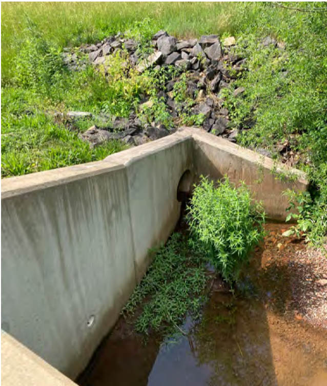
This culvert structure near the entrance drive directs an unnamed stream below Allentown Road toward the site.
