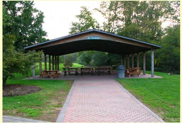
Beck's Pavilion– Beck's is also a new Cedar Forest pavilion that is in excellent condition. It is slightly smaller, roughly 45 by 32 feet, with unit paver base and is outfitted with electric supply and eight picnic benches.
