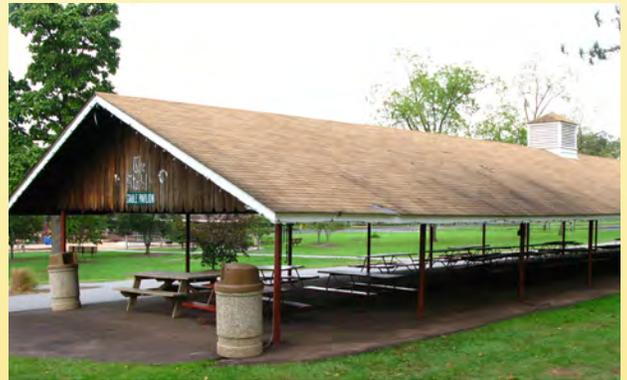
Carriage House Pavilion – This pavilion is located adjacent to 5-12 year-old playground. It is 22 by 80 feet and is in fair condition. The roof is older and the poured concrete floor is cracked. It is anticipated that this pavilion will be demolished if the Bustard Road Bridge is replaced and the road is realigned. The pavilion has roughly 10 unfixed picnic tables that are older but are in fair condition.
