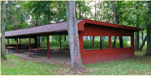
Boathouse Pavilion – The Boathouse Pavilion is located near Towamencin Creek in the 100-year floodplain. The roof contains holes and is in poor condition. The concrete floor is cracked and uneven. The picnic tables are old. This pavilion is note well used, is in poor condition, and should be demolished.
