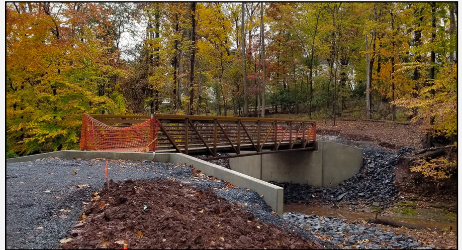
The recently installed pedestrian bridge along the new Kriebel Road Trail
