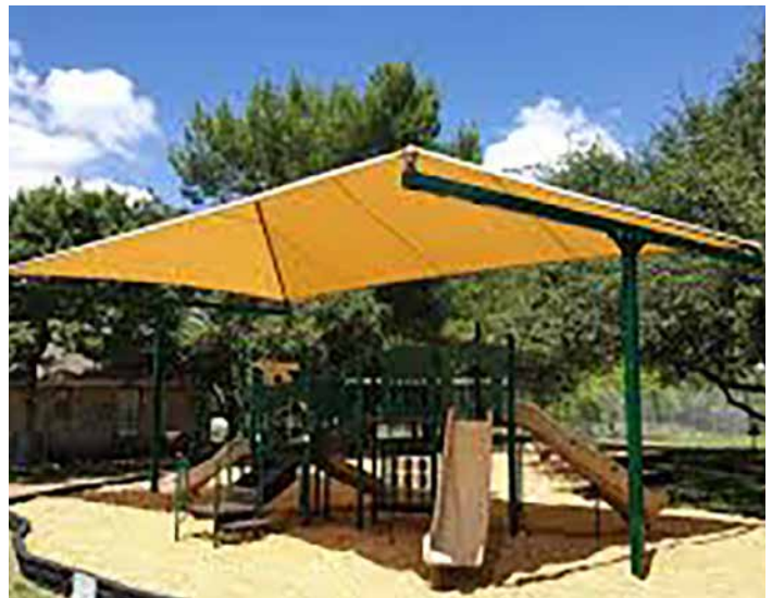
Playground shade structure. Photo from shadepro.com
