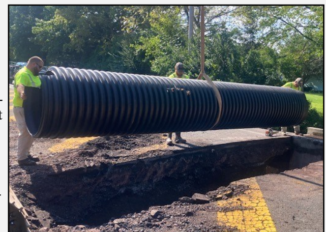
Public Works crew repairs sinkhole on Detwiler Rd. post Ida
