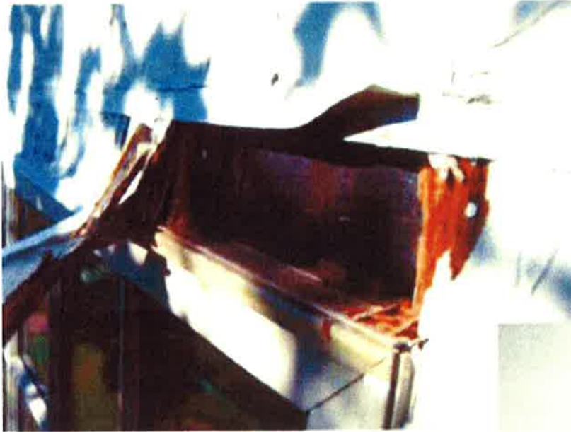
Typical Improper Flashing at Wood Junctions Flashing in front of Building Paper
