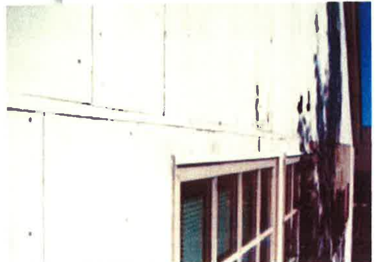
Typical Improper Flashing at Wood Junctions Flashing in front of Building Paper
