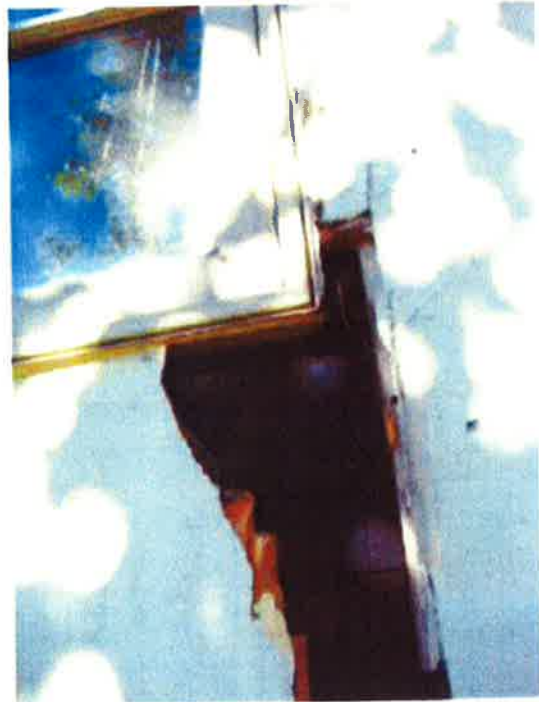
End Closure at Northea. Corner Never Installed
