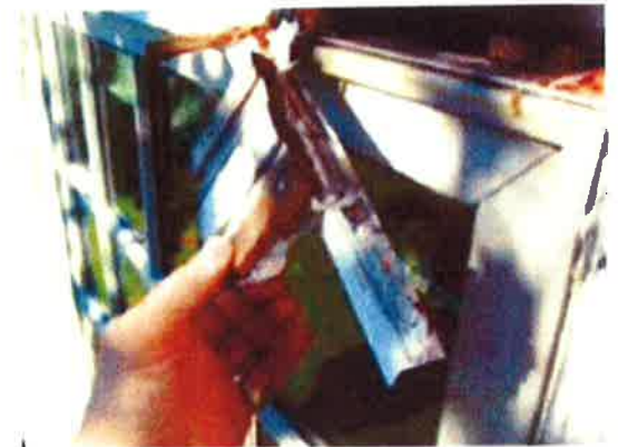
Demolition at Window Head Showing Typical Improper Flashing, Improper Caulking at Head Joints, Rotted Wood
