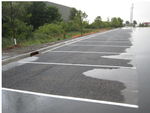
Porous pavement might be utilized in parking bays and walkways to contribute to on-site retention of stormwater.
