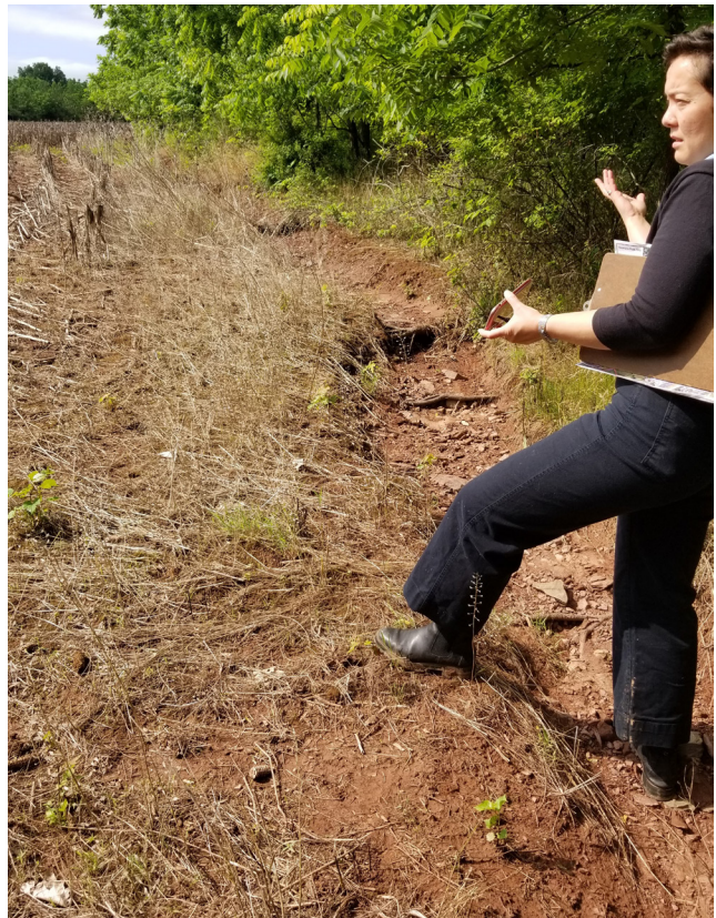
Eroded gullies are present along the western edge of the site (top) and through/around an outcropping of trees on the north side of the site (bottom).
