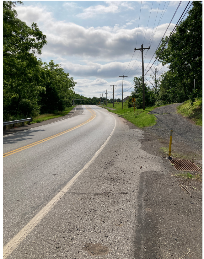
The only existing vehicular access drive enters the site from Allentown Road.
