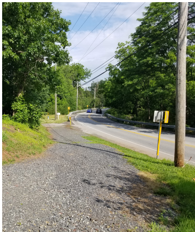
The existing entrance driveway is located at the apex of a curve on Allentown Road, and sight lines here are limited.
