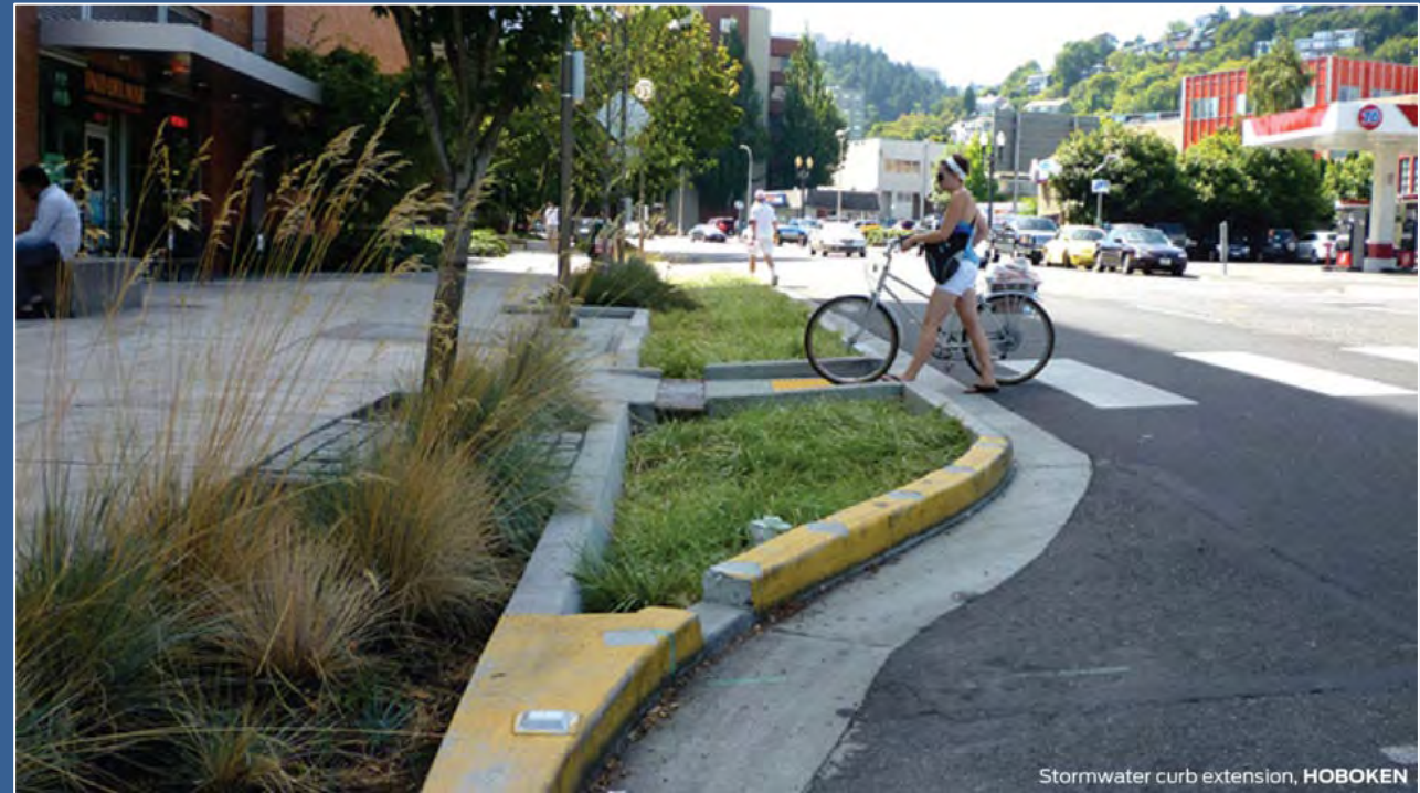
Stormwater curb extension, HOBOKEN
