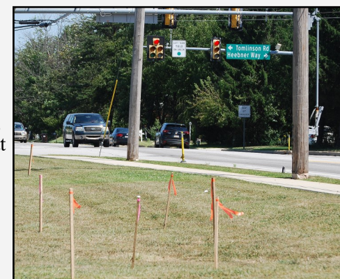
Stakes placed along Forty Foot Road, prepping for the widening project.
